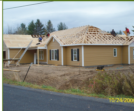
CARTHAGE, NEW YORK October 21, 22 and 23, 2009 GC: Olley's General Contractors, LLC
